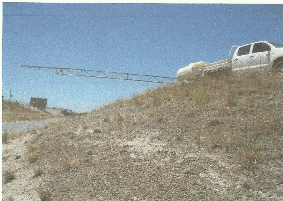
Figure 4. Boom spray emitting liquid gypsum on the harrowed channel batter.
